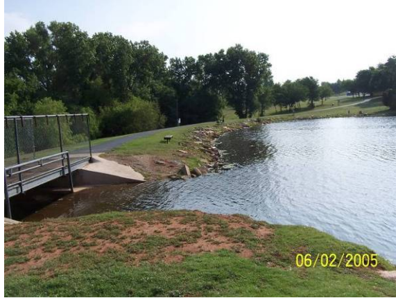
Figures 2 and 3: Concrete “Rip-Rap” on South and West Banks of Mulvey Pond
