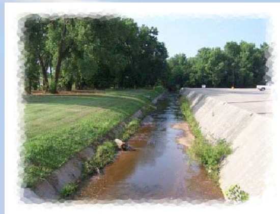
Typical hardened stream channel
